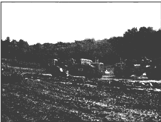
Figure 5. 12 Scraper hauling soil
