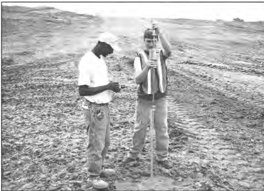
Figure 5. 6 Performing DCP a test
