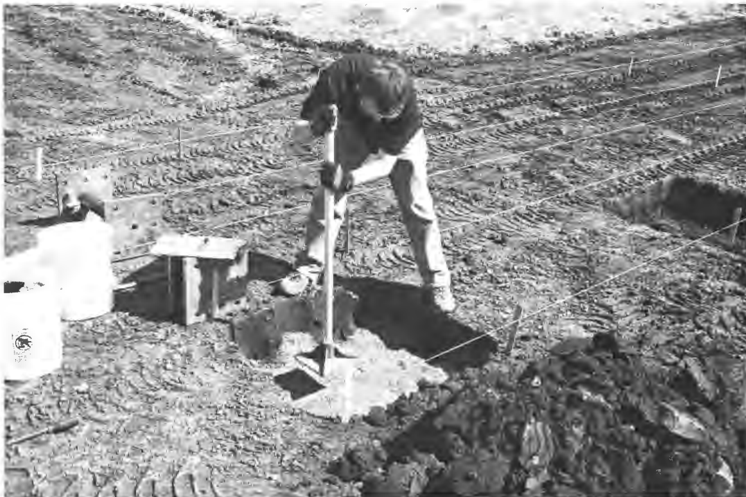
Figure 3. 10 Tamping the soil
